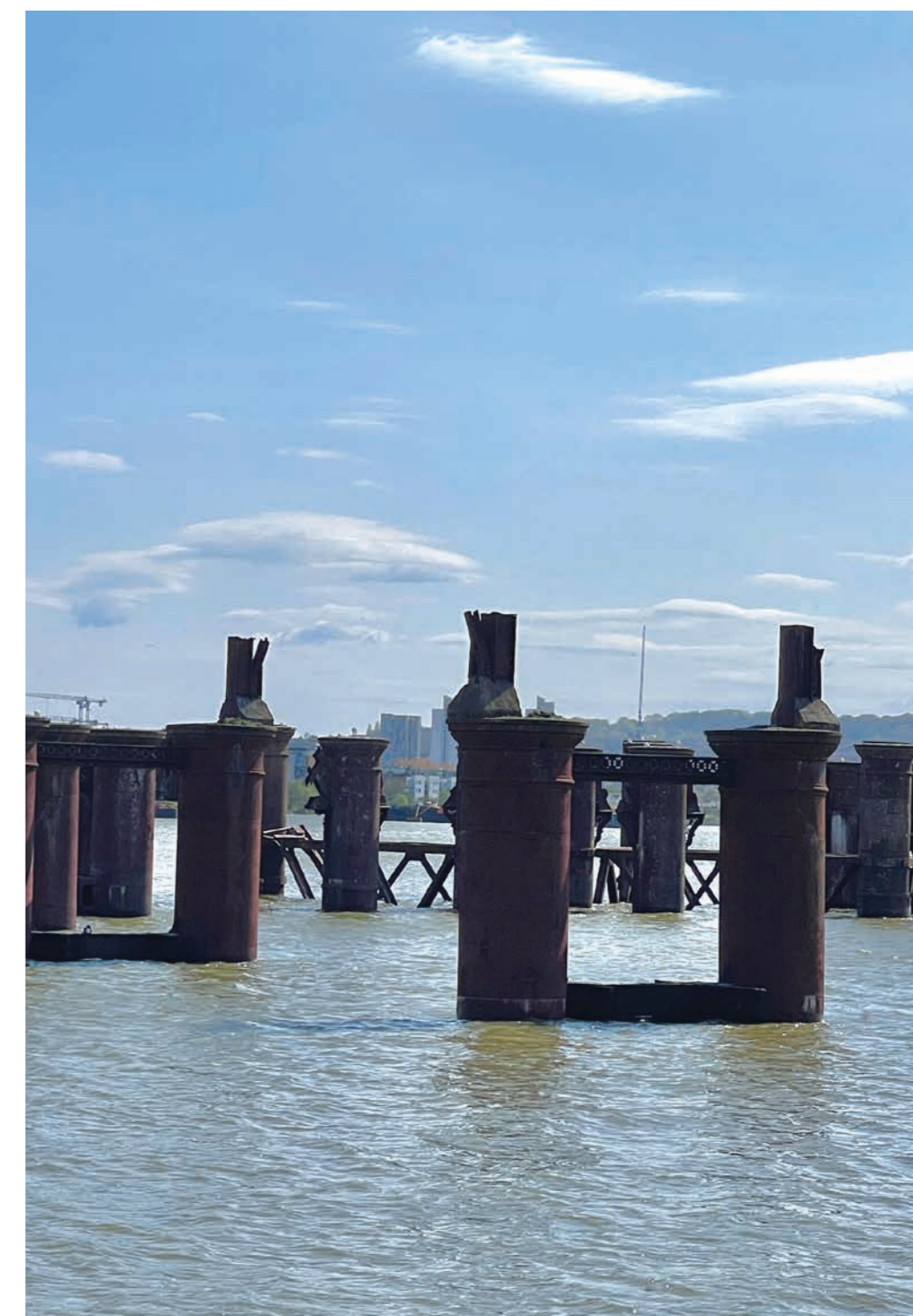
Disused Riverside Piers
